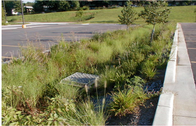
Figure 5. Parking Lot Bioretention Island
