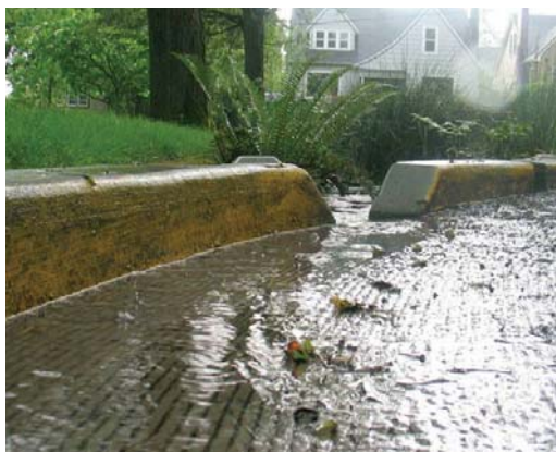
Curb Cut to Bioretention Cell
