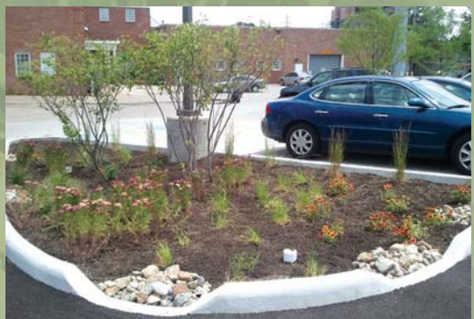
Bioretention Island with Trees for Shade
