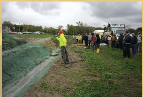
BMP Demonstration by Absolute Contracting, Inc.
