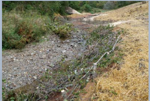
Streambank Stabilization at the Former Kenston Lake
