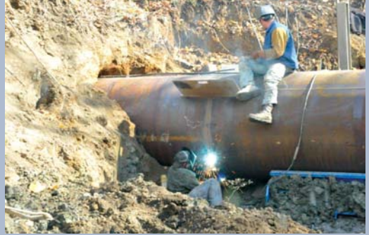
New Culvert Installation at Kenston Lake Dam
