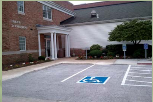
Permeable Concrete Parking Area
