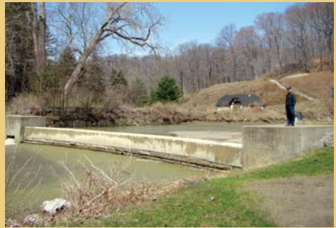
Dam on the East Branch
