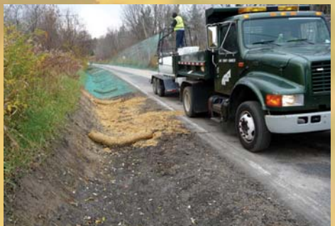
Straw Wattle and Hydroseed Mix Applied by Lake County Engineering Department
