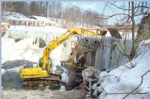
Drilling Weep Holes in IVEX Lower Dam
