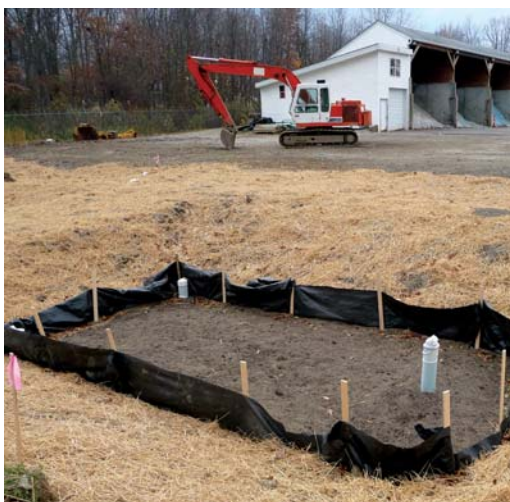
Concord Township Subsurface Gravel Wetland
