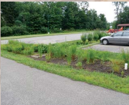
Bioretention Retrofit at Lake Metroparks Environmental Learning Center
