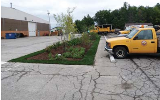
Eastlake Service Department Bioretention Cell Parking Lot Stormwater Retrofit
