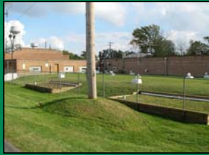
Bellwood, IL Water Department Rain Garden w native (class C) soil: 2.3" 24-hr storm
