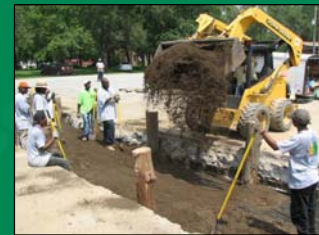
Chicago GreenCorps at Our Lady Gate of Heaven project site
