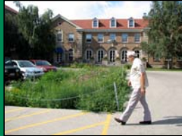
St. Margaret Mary Bioswale w. amended soil over sandy soil: 6+" 24-hour storm
